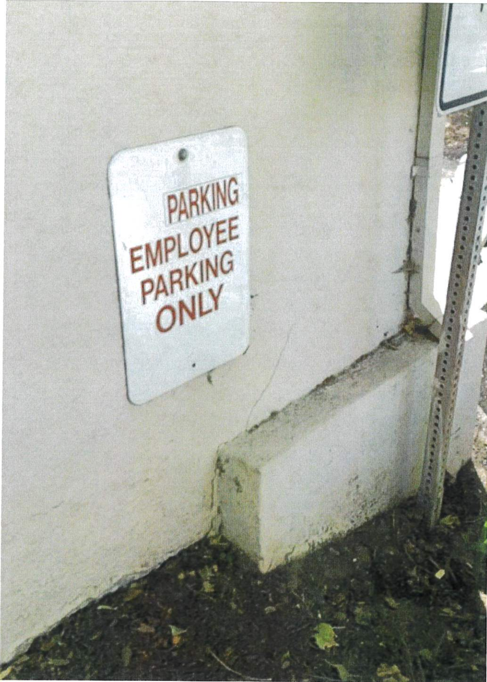
Photo 2 – Crack in Exterior Wall
